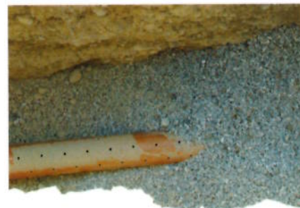
Installation of the drainage system at the on-farm demonstration site at Rumais, Oman. Barley was planted on this site in December
